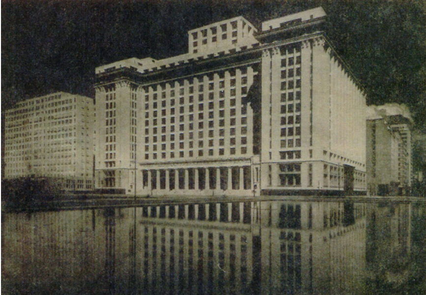
FIGURE 3 The Palácio do Trabalho building in stripped classical style, and, on the left, the headquarters of the Ministry of Finance (1944).
